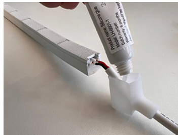
7. Fill end cap with one layer neutral-cure silicon
